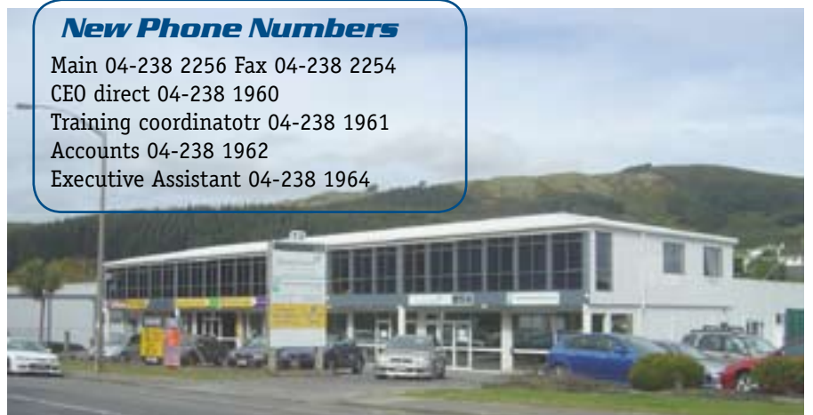
The view of the new first-floor premises coming north from Tawa.
